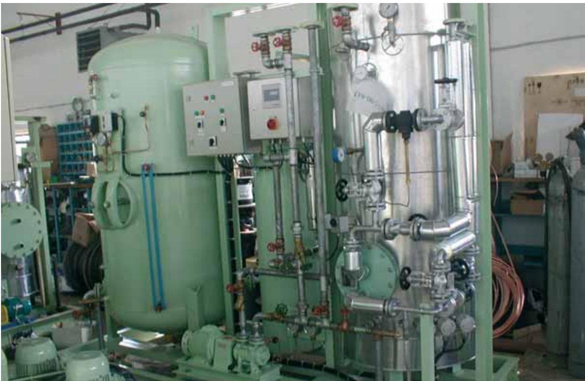
Compact units consisting of hydrophore, filter, sterilization and calorifer
